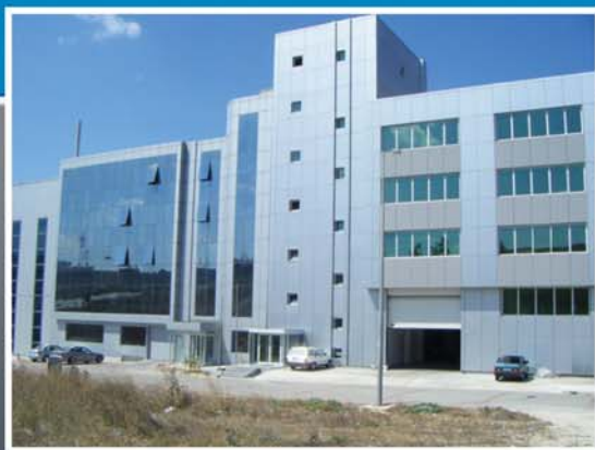
TouchIT Technologies manufacturing facility, Istanbul, Turkey
